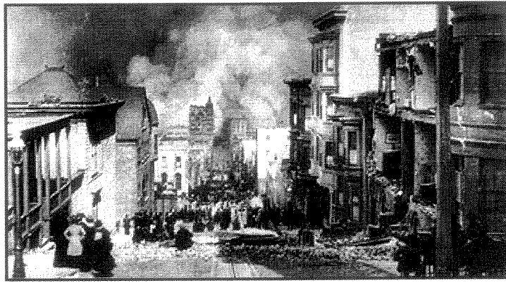
The great 1906 San Francisco earthquake and fire destroyed most of the city and left 250,00 people homeless. Full size image - 151k.
